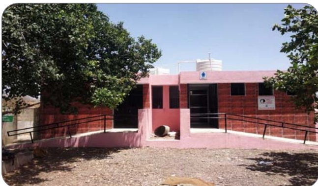
Renovation of School Sanitation unit at Dwarka, Gujarat
